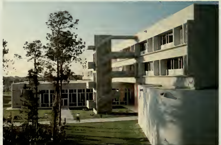
Stair towers express themselves by pulling away from the building. Photograph: Hedrieh Blessing/Nick Merrick
